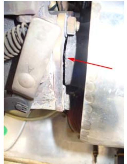
Figure 15: Crack in 914 exhaust pipe.
