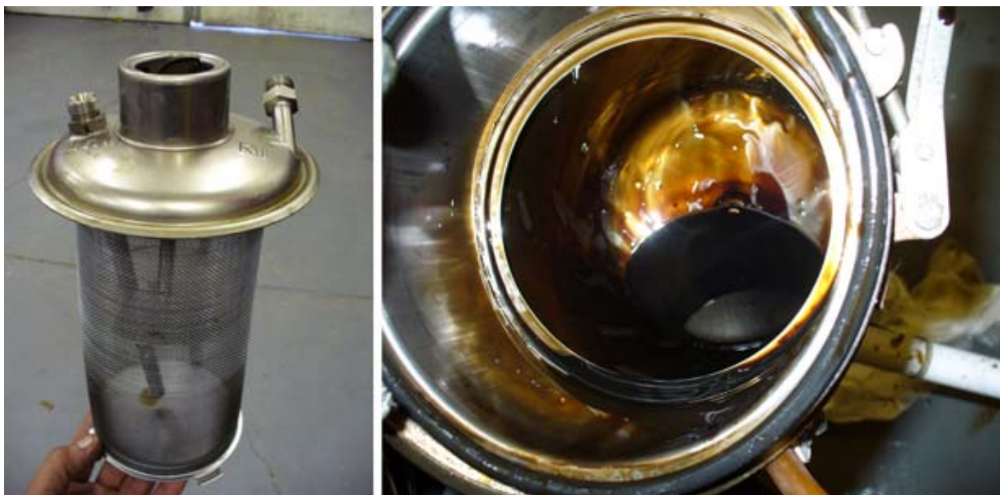
Figure 10: Dismantled oil tank
